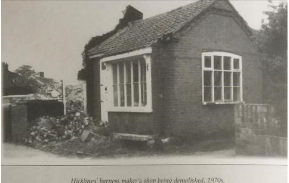
Hicklings' harness maker's shop being demolished, 1970s.
