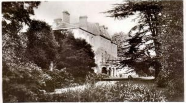
Ryston Hall by WHS Kingsway.
