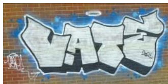
Graffiti attack on Hethersett Village Hall.
