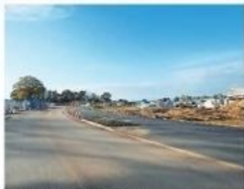
New houses being built in the north of Hethersett
