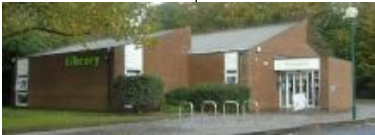
Hethersett Library—the present venue for the temporary pop up post office.
